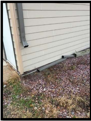
Northeast Corner – Completely disconnected.
