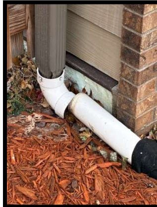
Northeast Corner – Completely disconnected.
